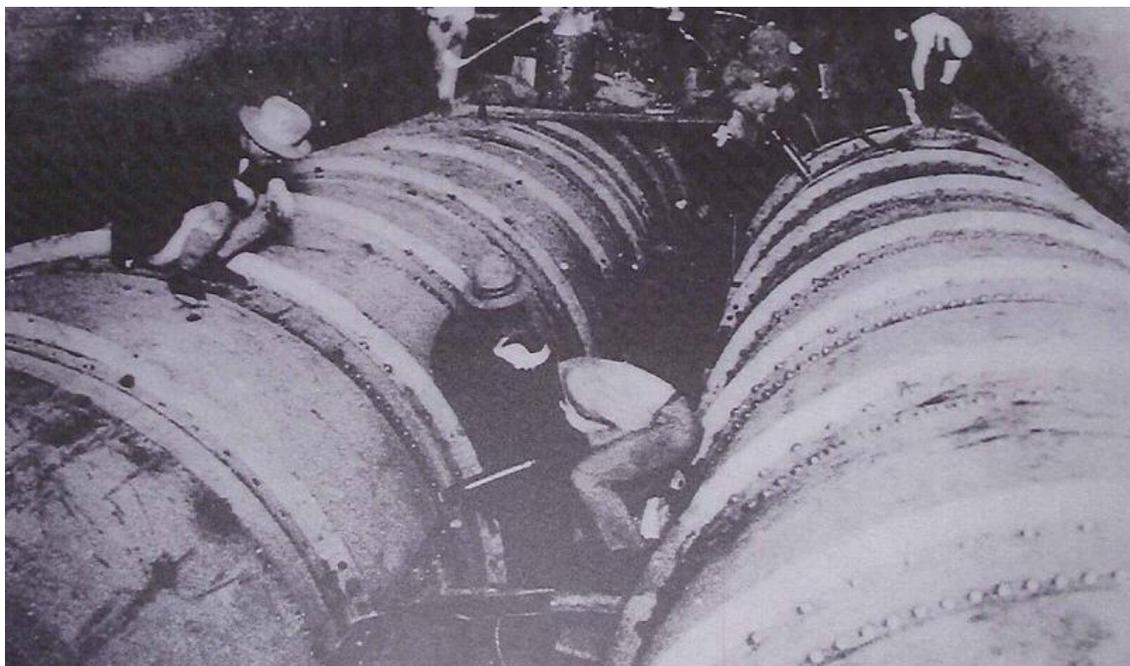
**Figure 13:** Riveting work for the iron pipes connecting the Sonnun-kei river with the Kandem-kei river to fill the water in the Uzanto-dam lake.
