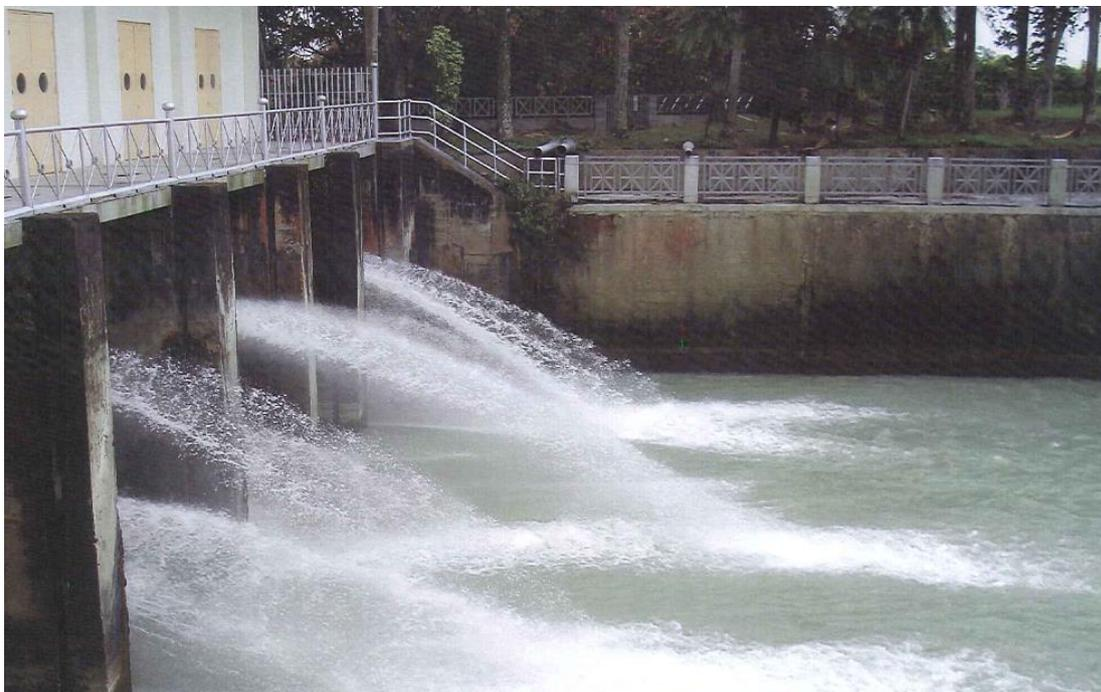
**Figure 11:** Discharge from the conduit exit through the Uzanto-dam bank.
